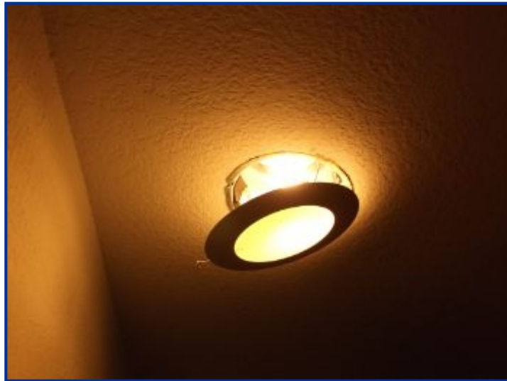
Fixture in upper front left bedroom
