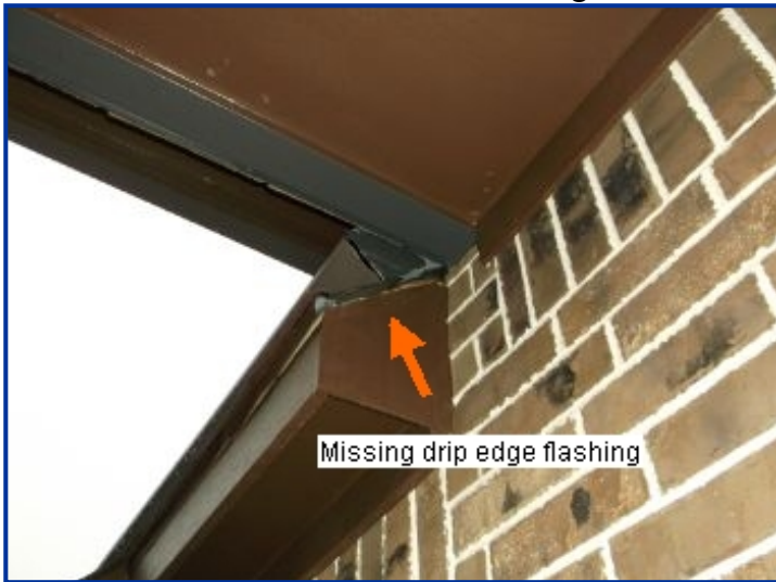
Roofing eyebrow over exterior door between garages
