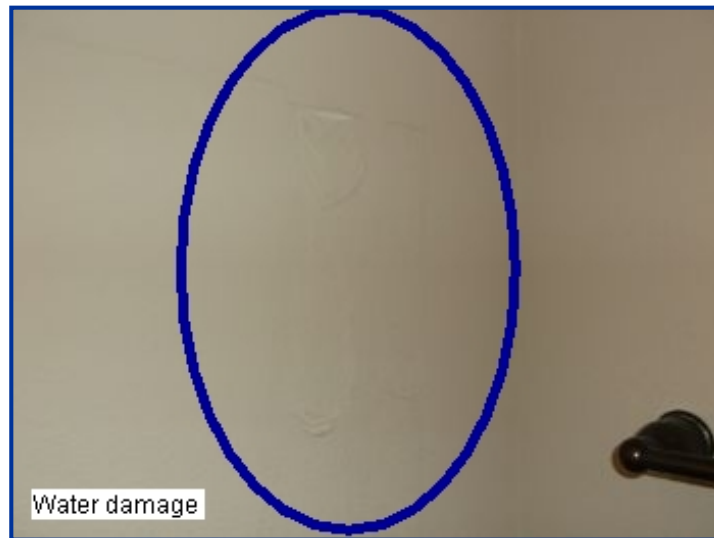
Wall over commode in lower left bath
