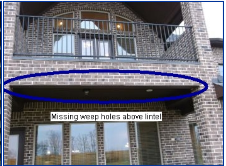
Masonry beneath upper rear porch
