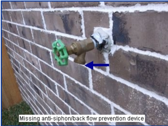
Left elevation hose bib
