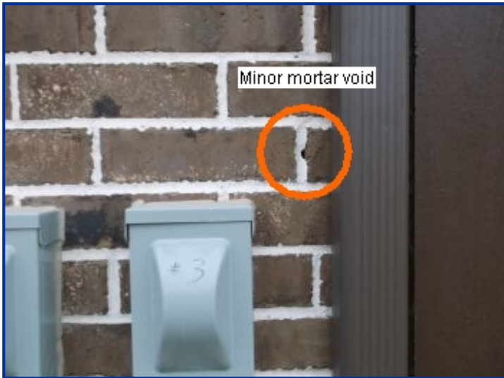
Right elevation masonry wall near A/C disconnects
