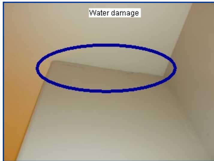
Ceiling above commode in lower left hall bath
