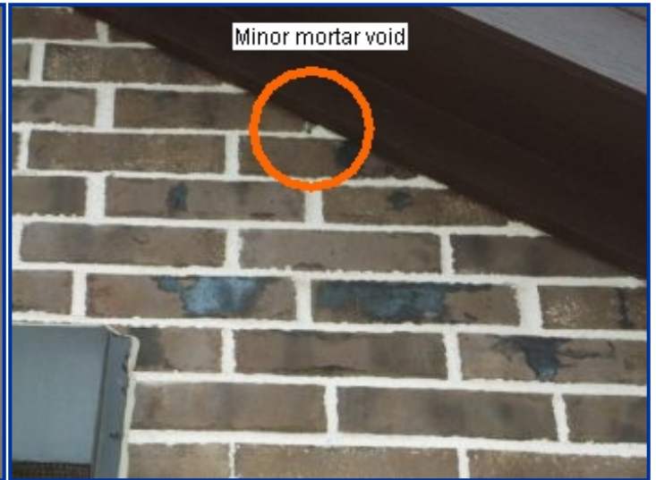
Right elevation over A/C compressors
