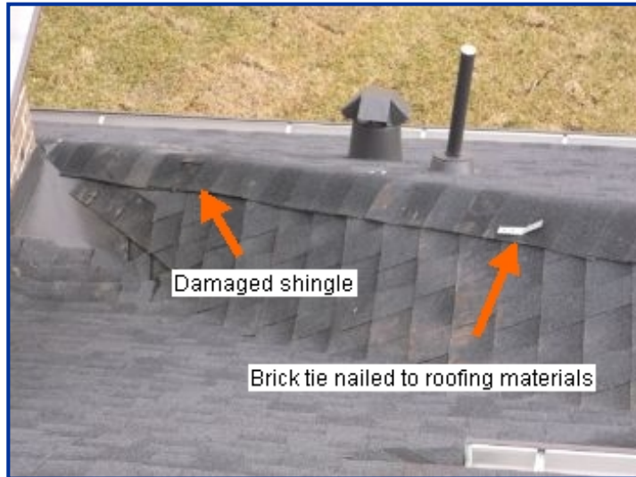
Lower left elevation roofing application
