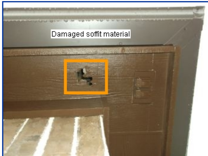
Left forward soffit corner
