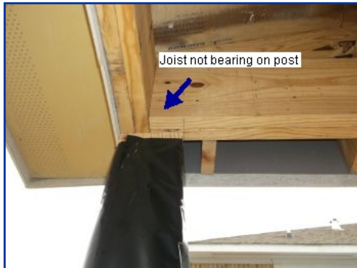
Front porch (left post)
