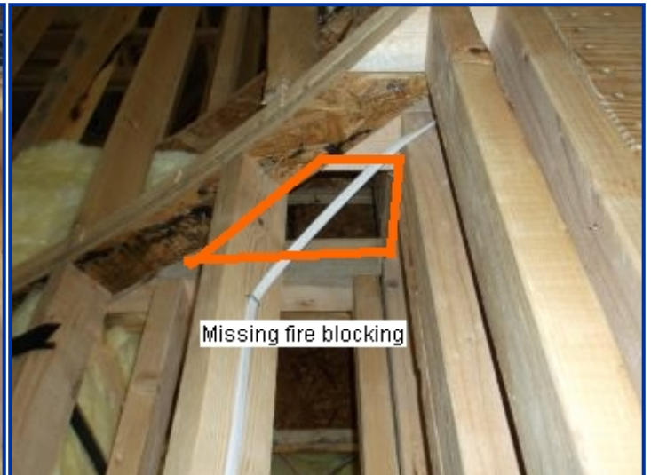
Chase at base of stairs
