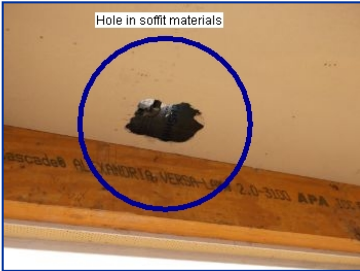
Rear porch ceiling
