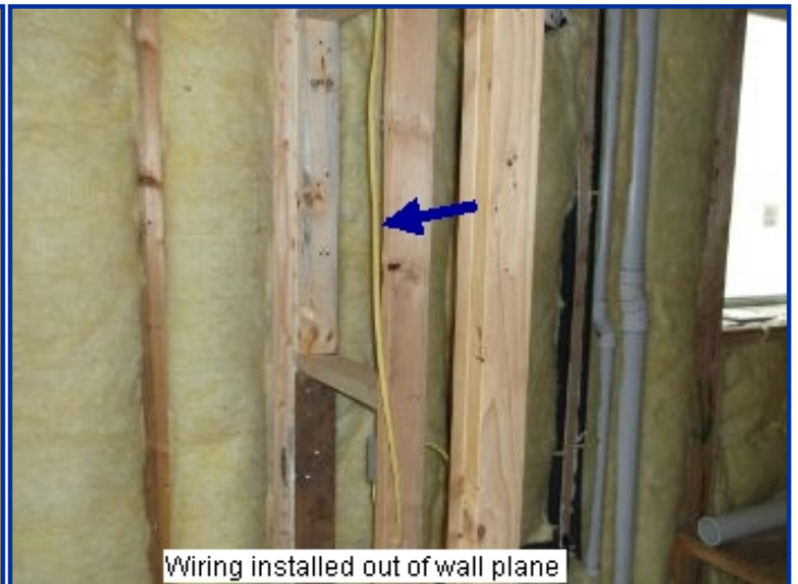
Master bath rear sink area (medicine cabinet framing)
