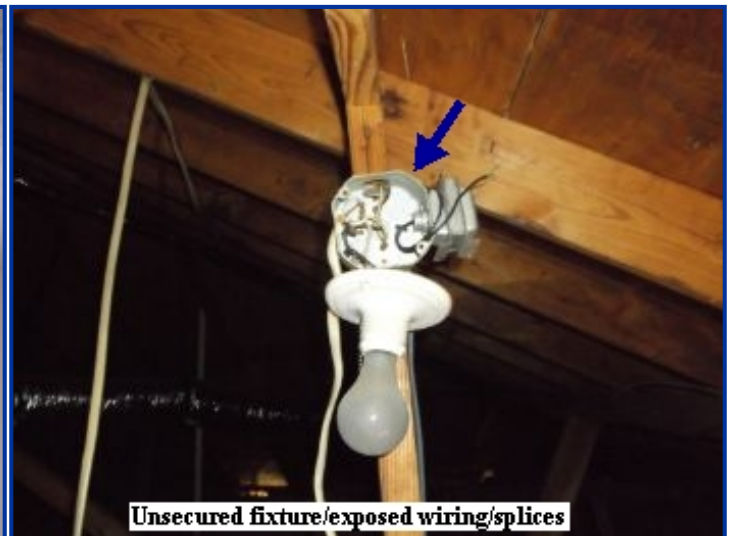
Exposed bulb fixture
