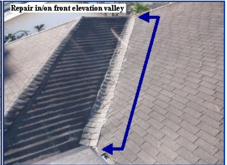
Roofing application (repair)
