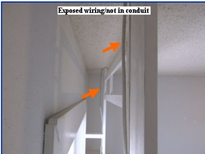
Exposed wiring/not in conduit
