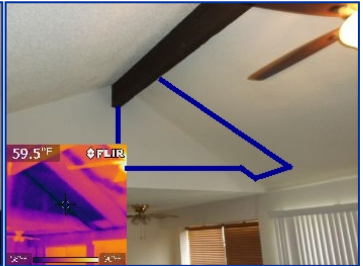
Living room (left) rear upper wall/ceiling
