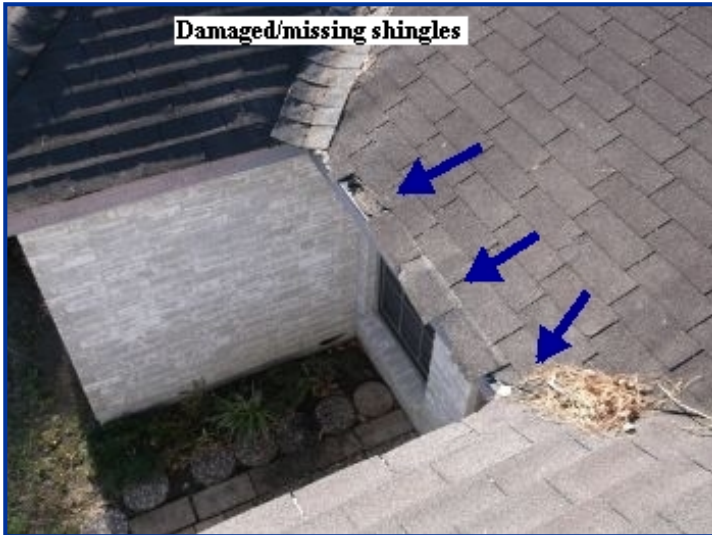
Front elevation roofing application
