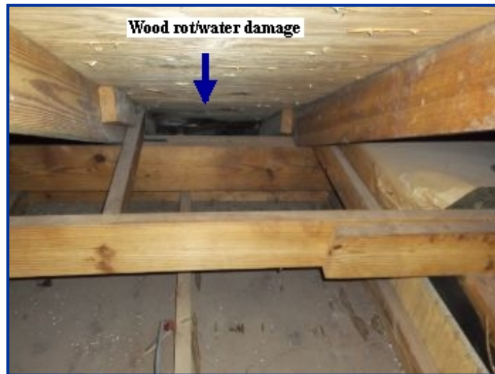
Decking at eave above front porch
